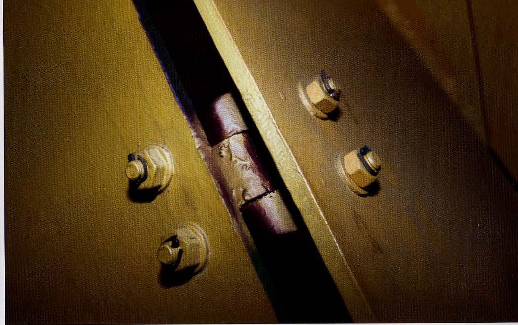
The upper hinge was secured with four bolts on the inner surface of the rear plate and the door. Two hinges were attached for each door.
